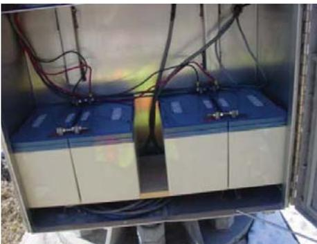
Figure 1: AGM batteries in a cabinet for Wavetronix Sensor
