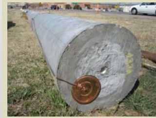
A concrete camera pole ready for installation.
