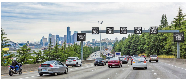
Figure 2. Photo. Variable message signs showing traffic alerts and speed limits for individual lanes.
