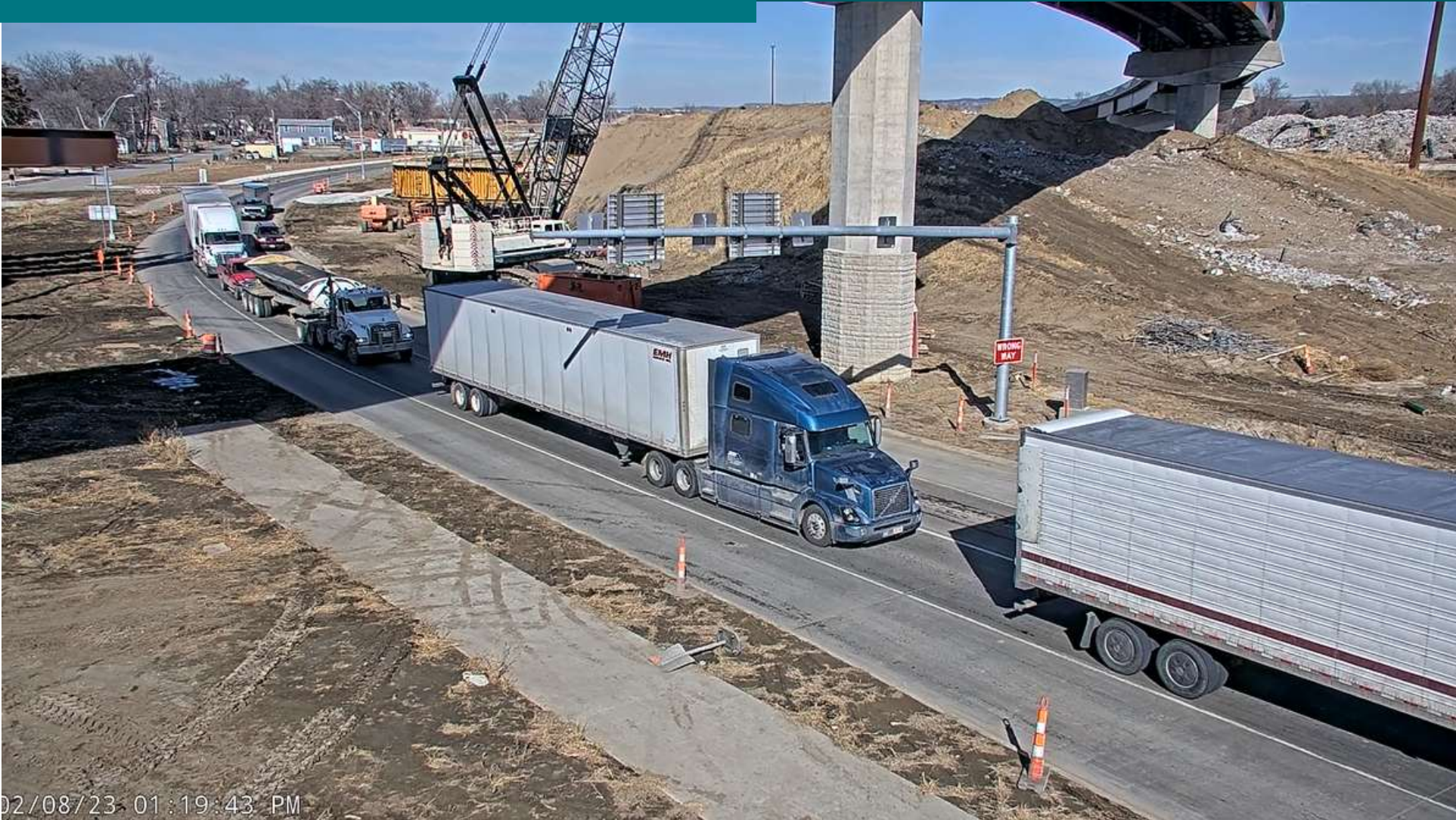
SB Frontage Rd at Broadway (looking north)
