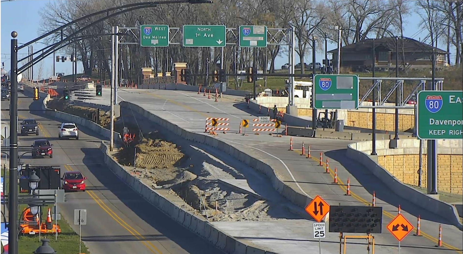
Tuesday 11/13/2023 – 8:50 AM Traffic Control Switch to Phase 3 Note 6' Grade Difference
