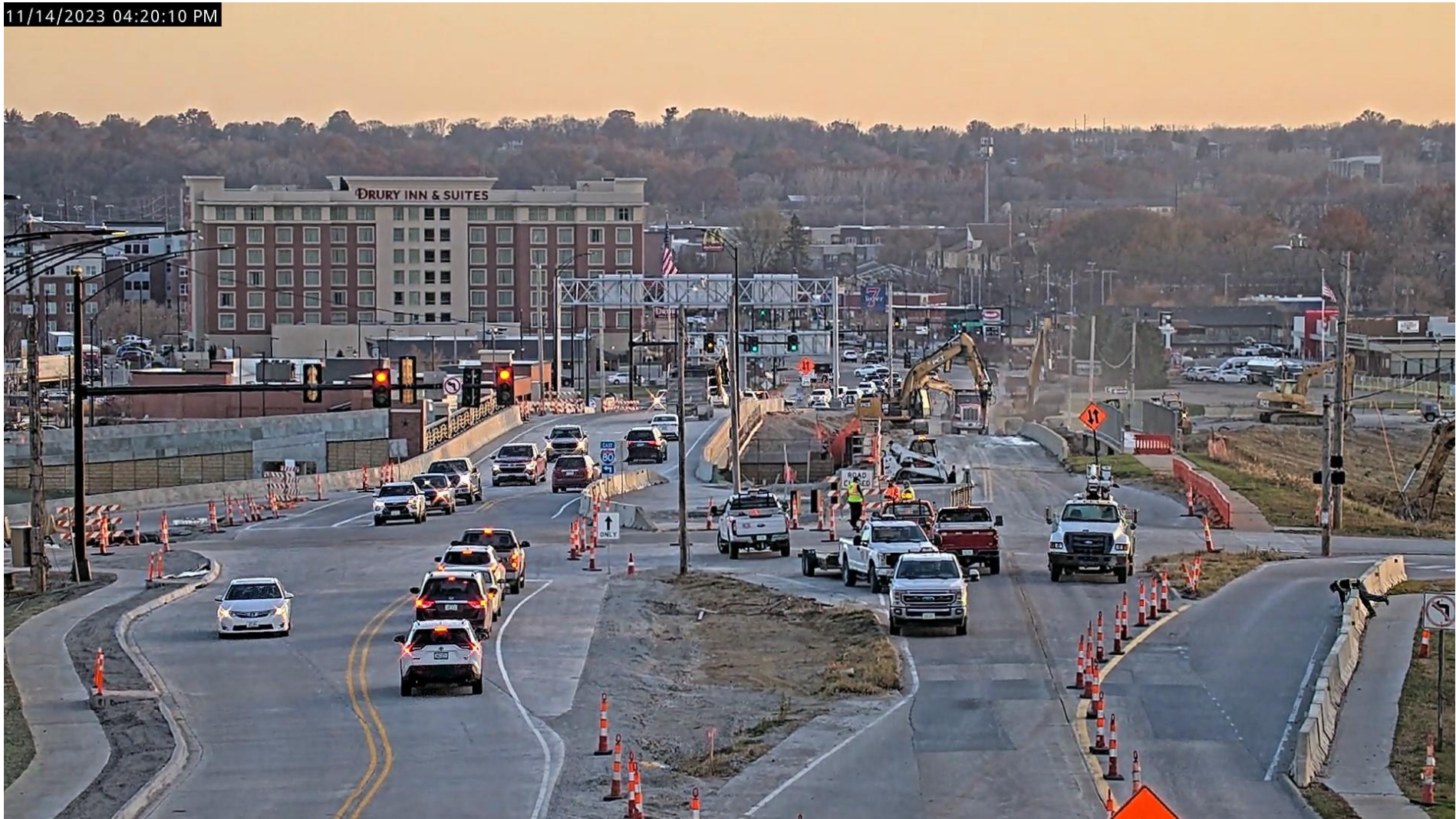
Tuesday 11/14/2023 – 4:20 PM Removal of West Bridge!!
